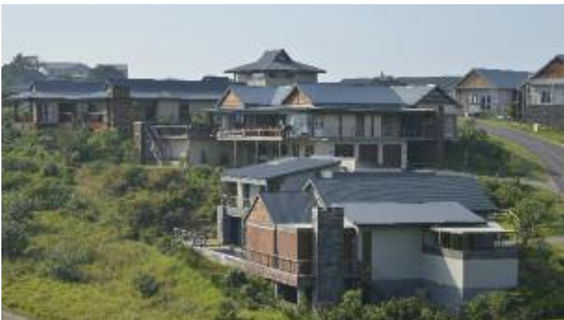
RESIDENTIAL DEVELOPMENT (750 houses in an estate in KwaZulu-Natal)
